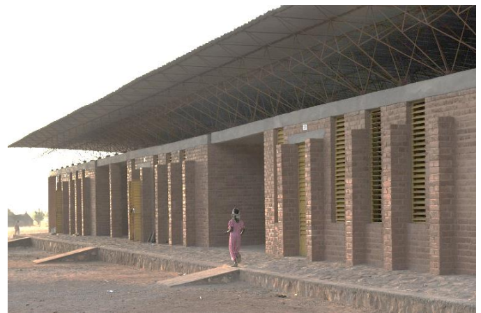
Figure 3. Gando school, illustrating the overhanging tin roof. Courtesy of Architecture Review.
